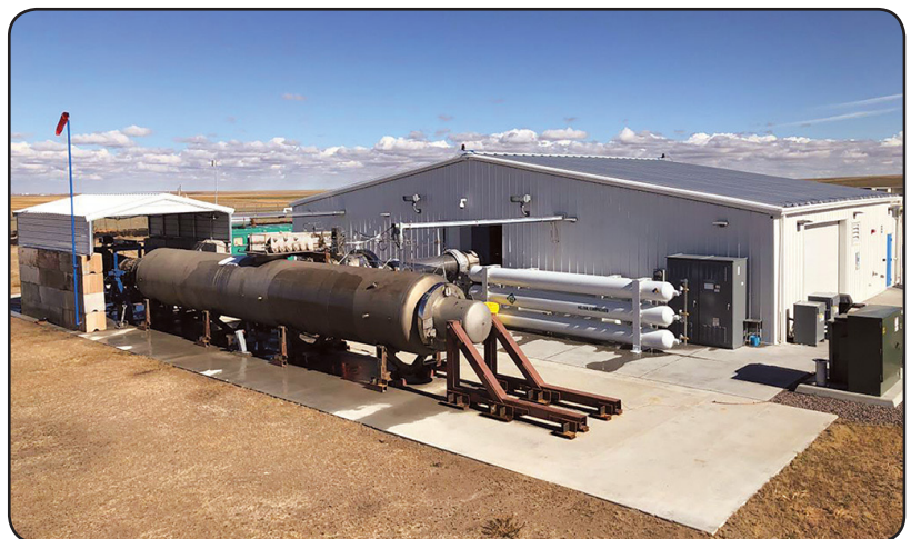
Heated air mass from the GE J79 under the cover (left), is conditioned by the plenum (center) before being ducted to the pre-cooler in the building.
